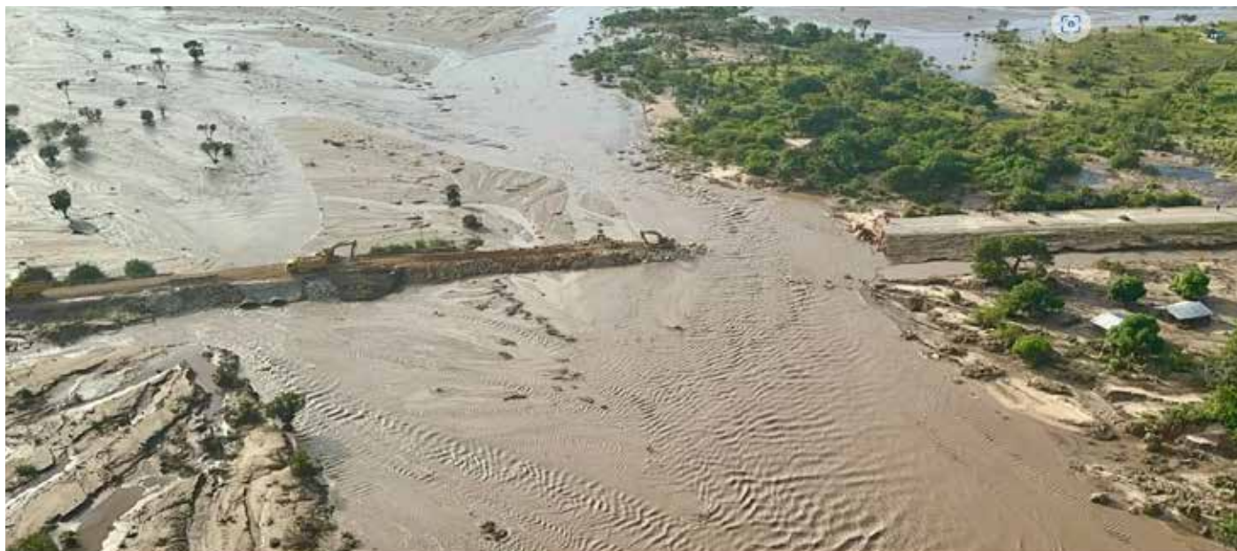
Figure 12: Aerial survey indicating the extent of damage of Lindi-Dar es Salaam Road after the landfall of the Tropical Cyclone Hidaya on 4 th May 2024. Source: Tanzania Media of 7 May 2024, accessed online on 5 th Feb 2025 at https://tanzania.eu.com/aerial-survey-of-lindi-dar-es-salaam-road-after-typhoon-hidaya/ .
